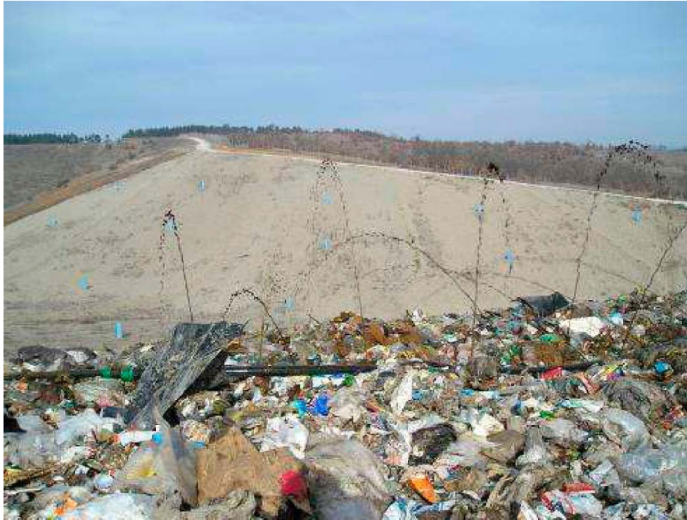
Fig. 55. Example of recirculation of leachate in Gjilan / Kosovo (Serbia, presently administered by UN ): Acceptable practice only if the alternative would be to release the leachate into ground or surface water. More appropriate (due e.g. to aesthetic and health aspects): would be to recirculate it under a covered landfill area with a proper gas collection system operated in parallel.
