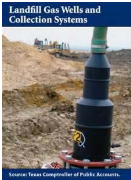
Fig.5. Landfill gas is extracted and piped to a main collection header, where it is sent to be treated or flared.
