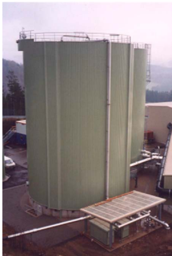
Fig. 49. Digestion facility for biowaste with biogas-engine
