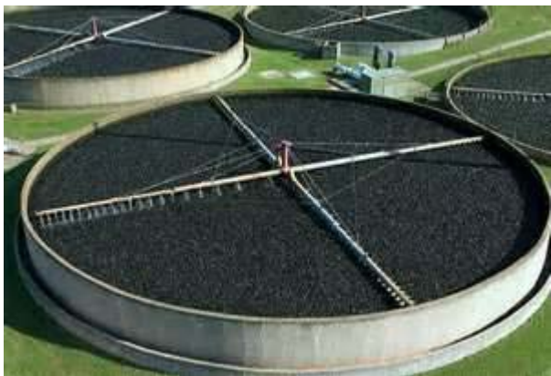
Fig.46.Trickling filter, sewage-treatment plant, Henderson, USA
