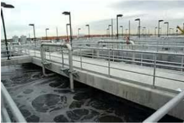
Fig.47.Activated sludge aeration basins
